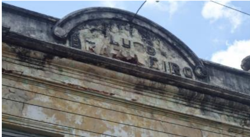
Figure 3: Part of the façade with sign of the Hotel Luso Brasileiro
