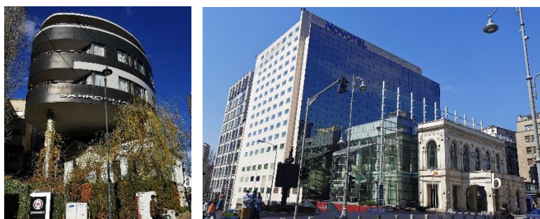
Figure 5 a, b. Modern hotels built in the protected built-up areas being in contrast with the traditional urban fabric generating a visual pollution. Source: Merciu G.-L.
