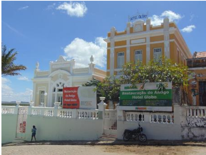
Figure 6: Hotel Globo under restoration
